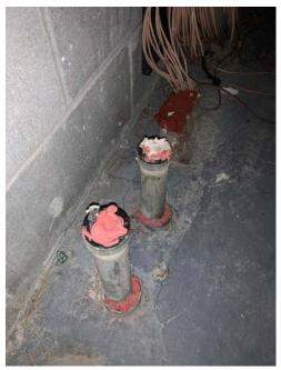
Photo 15 & 16: Asbestos-Containing Spray On Fireproofing Debris on Floor, Conduit and Walls – Ground Floor – 7<sup>th</sup> Floor (Electrical Closets)
