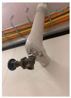
Photo 28 & 29: Asbestos-Containing Job-Molded Plaster Pipe Fitting Insulation – Throughout Basement & Ground Floor
