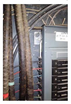
Photo 11 & 12: Asbestos-Containing Spray On Fireproofing Overspray/Debris inside Electrical Panel Boxes – Ground – 7<sup>th</sup> Floor (Electrical Closets)
